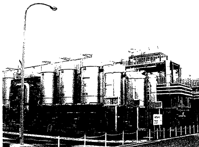
FIGURE 2.16 The 11-MW plant in Goi, Japan based on PC-23. The fuel cells are contained in the upright cylindrical vessels. (Courtesy of UTC Fuel Cells.)
